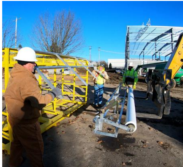
Insert the guardrails.
